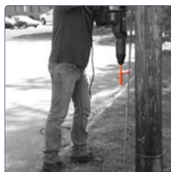
Drive the rod down to a comfortable height
