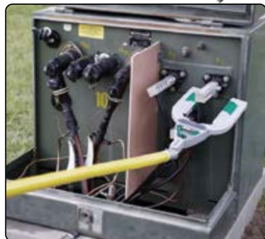
8-024PLUS Wide Jaw shown on Pad-mounted Transformer
