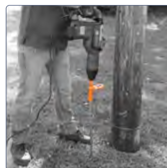
Then complete the driving by hammering from the top
