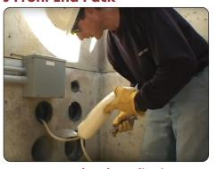
**Front End Pack Application** Demonstration of how the Front End Pack is used to assist conduit lubrication
