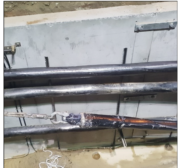
Cable Lube on completion of pull
