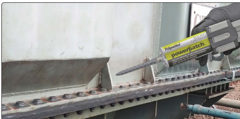
Major Substation Leaking Transformer Repair
