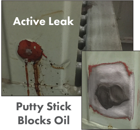
Repaired Leak
