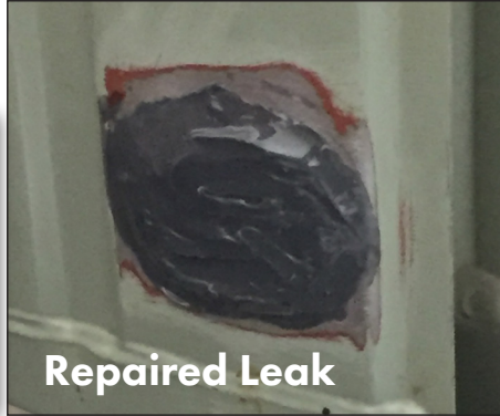
Apply with standard Caulking Gun
