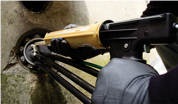
FST Sealant Pumped into Duct
